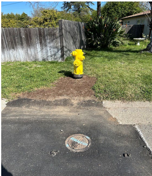
(New 6" wet barrel hydrant on Francis Way)
