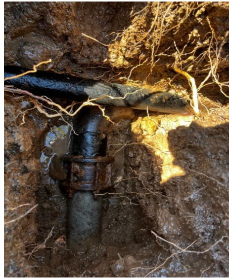
(Abandoned 4" Steel water main)
