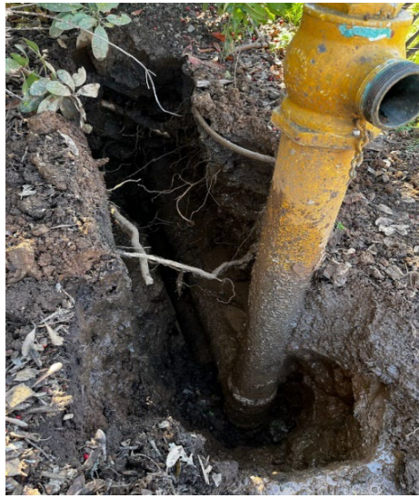
(Removed 4" Steel wharf hydrant)
