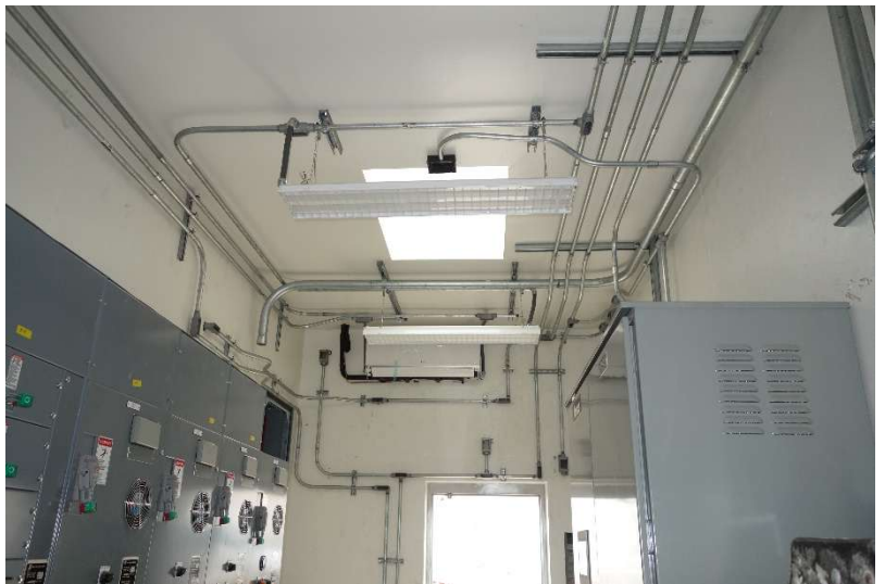
Electrical Room Conduits/Lights A/C
